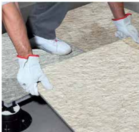
INSTALLED AS A FLOATING FLOOR
