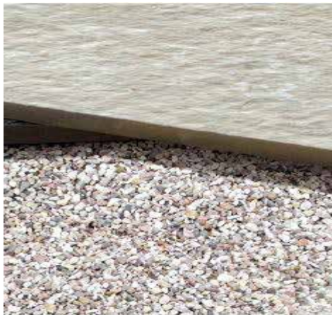
LAYING OVER SAND
