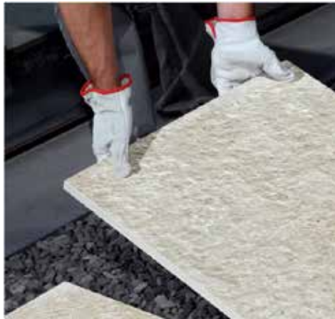
LAYING OVER GRAVEL
